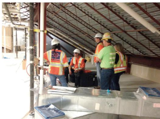
One of the engineers on the project suggested aeroSeal. This would allow the contractors to easily seal the 48 shafts running throughout the 88,000 sq ft building. It would not require any demolition of existing walls and the process would automatically provide results data.
