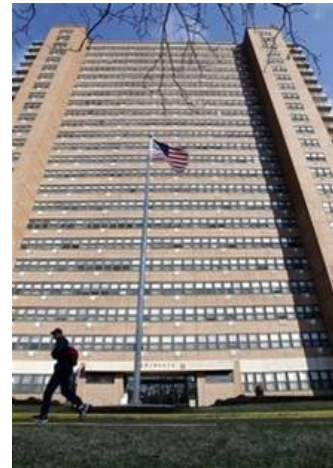
Northgate II low-income high-rise reduced utility costs $37,000/year by effectively sealing leaks in its 29 exhaust shafts
