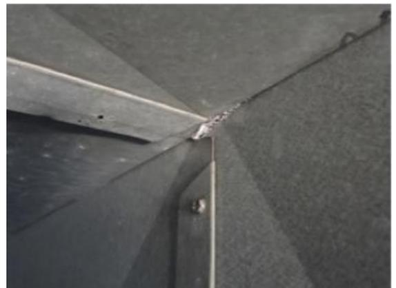
The sealant doesn't coat the duct interior but accumulates primarily in and around the leaks.
